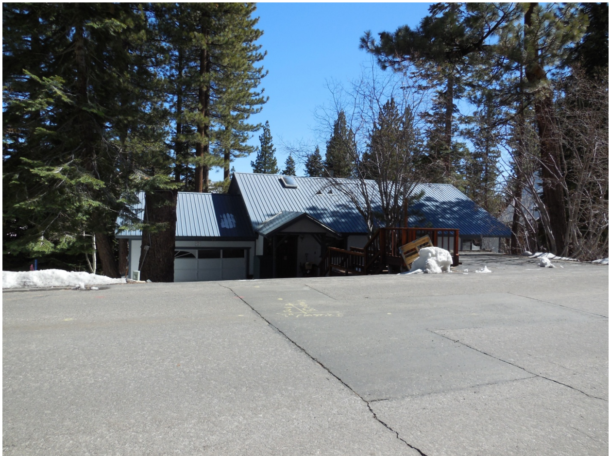
View of the garage and house from the street.
