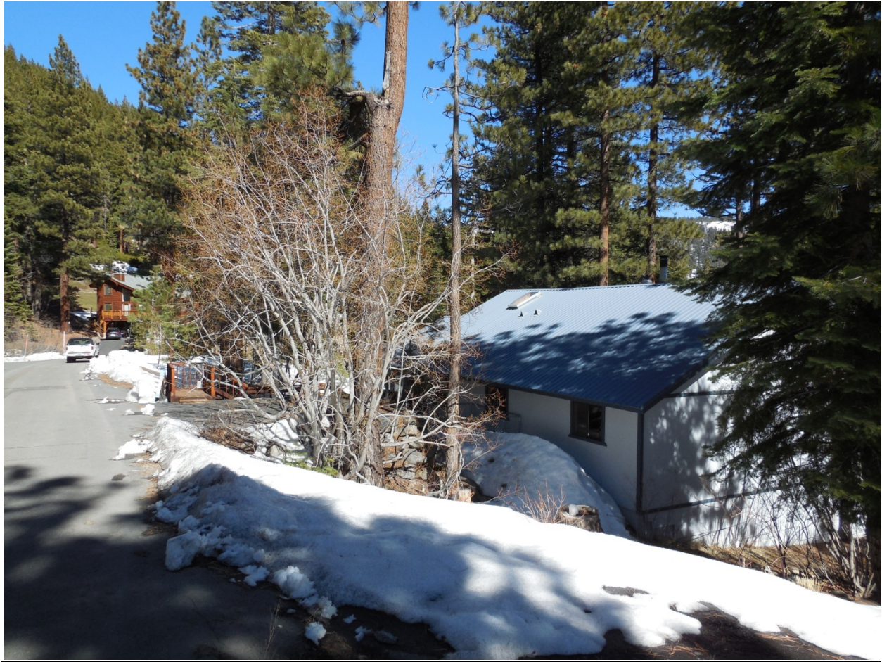
View of south side of house. The floor level of the house and garage are far below the street.
